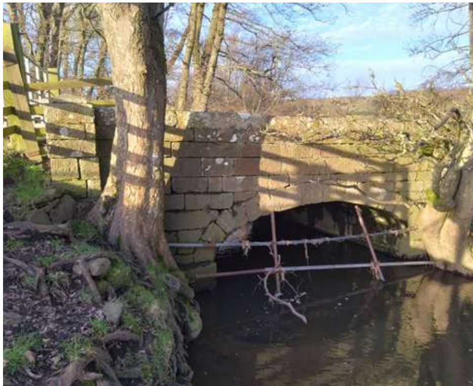
PG 02 - Bridge Carrying Drive To Greencroft Park Over Newhouse Burn (NHLE ref. 1116302)
