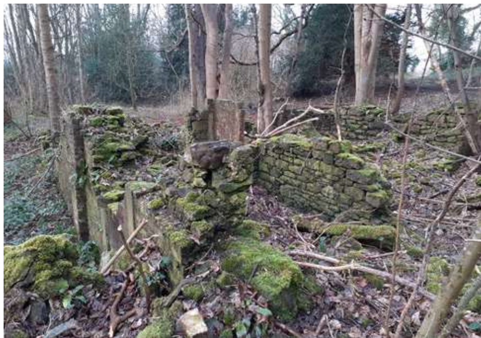
PG 16 - Former buildings at northern corner of the walled garden, looking south-west
