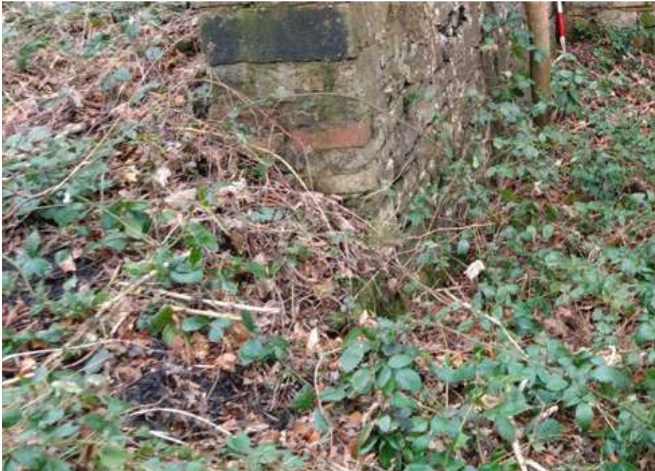
PG 22 - Former mine-entrance in Shoulder of Mutton woods, looking north-east
