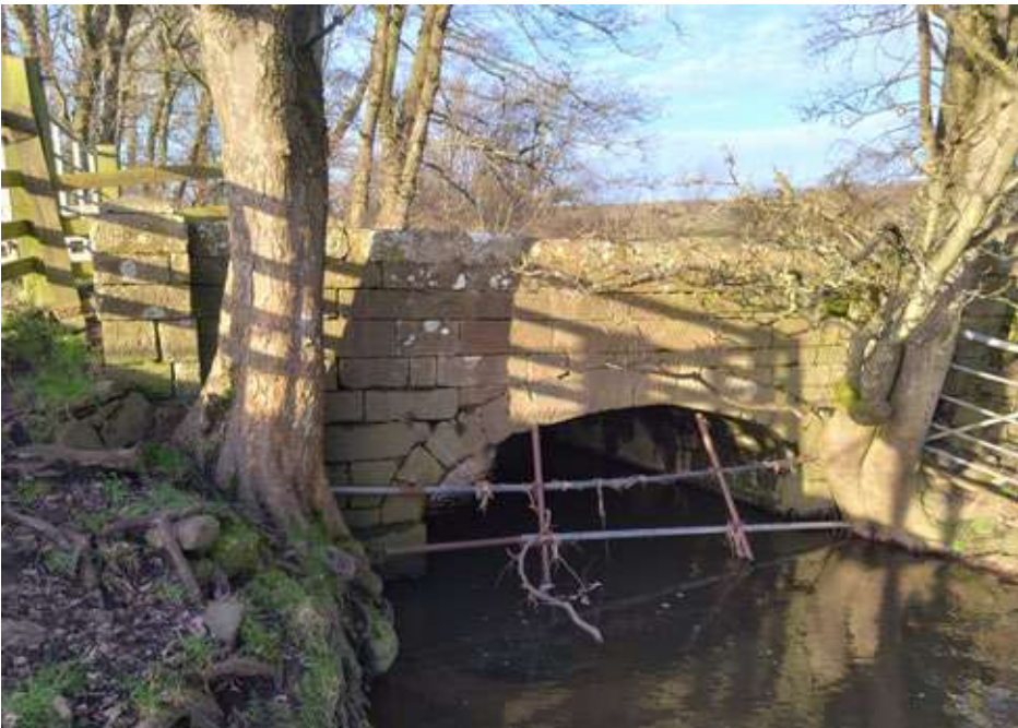
PG 12 - Grade II Listed bridge on Low Town Lane, looking north
