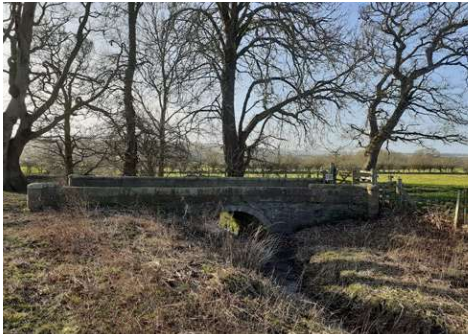
PG 11 - Unlisted bridge over Howden Burn, looking south-west
