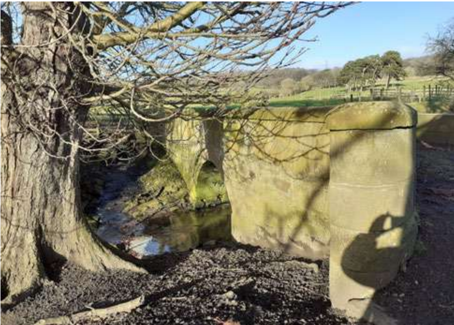
PG 10 - Unlisted bridge over Howden Burn, looking north
