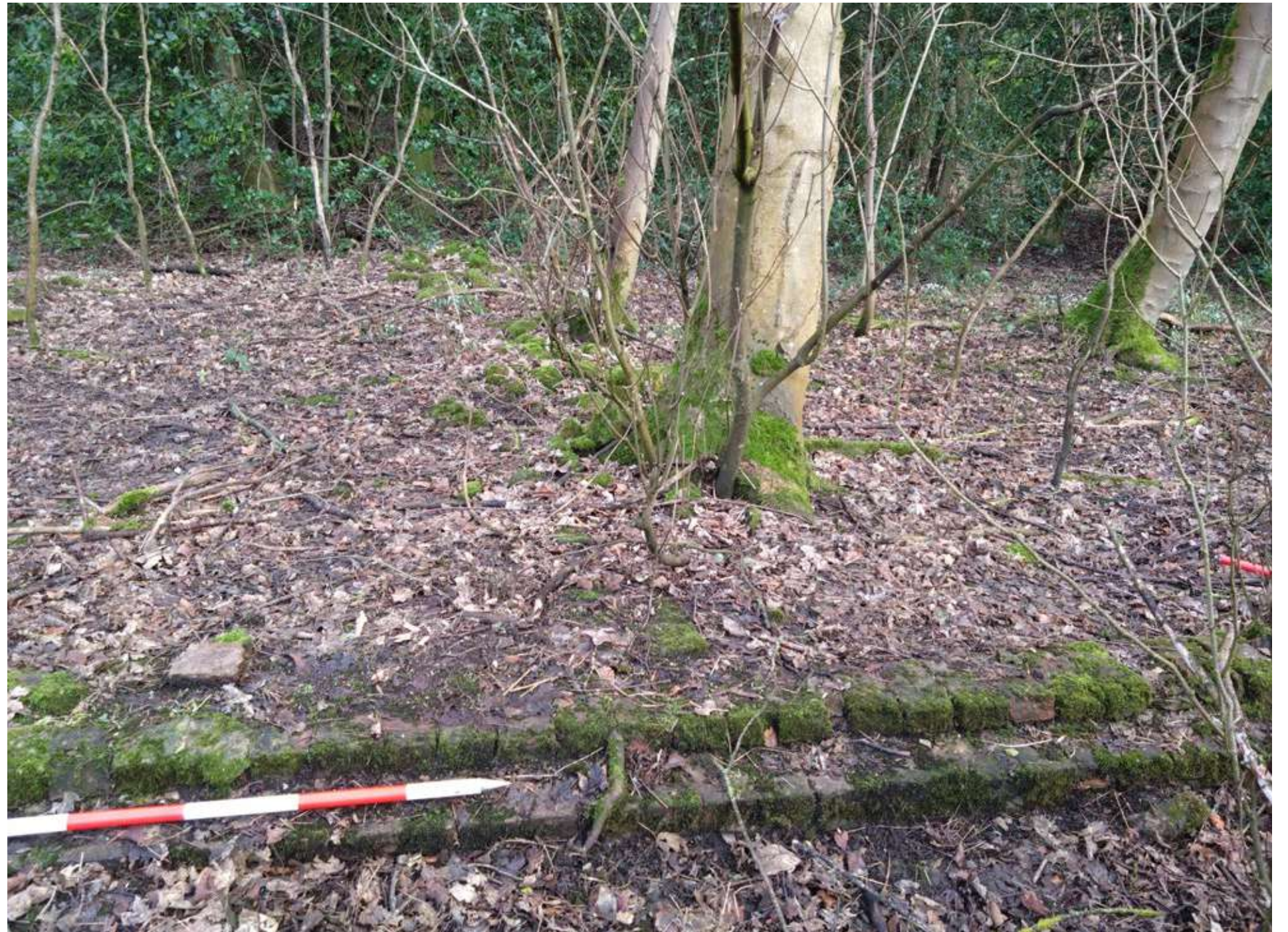
PG 17 - Garden wall footings, looking north-east
