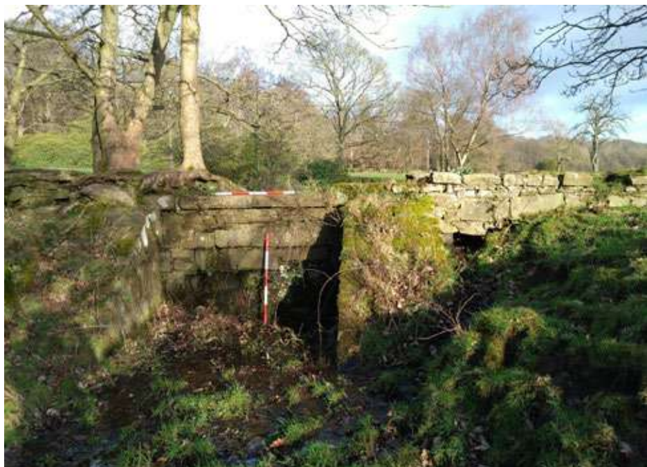
PG 07 - West end of pond, revetment and channel, looking north-east
