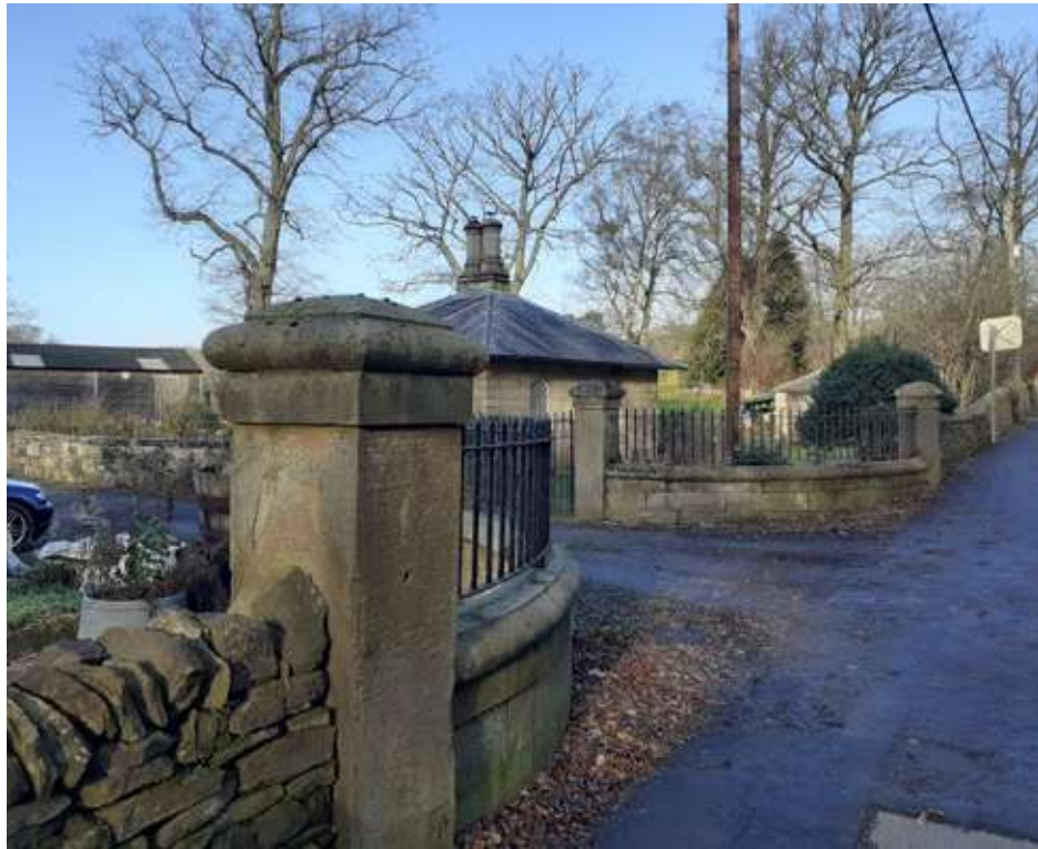
PG 01 - Piers And Walls South East Of Fenhall Lodge (NHLE ref. 1185966), looking north
