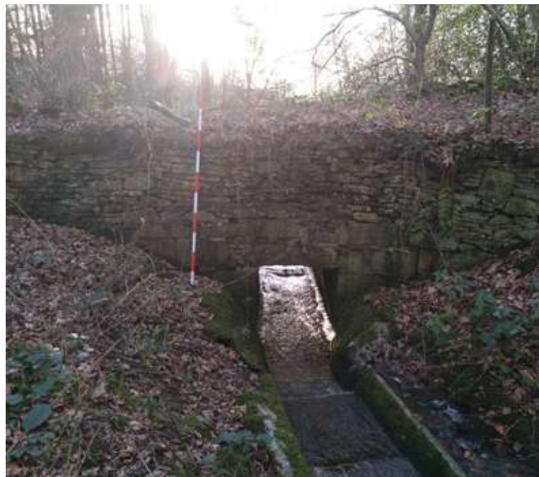
PG 26 - Causeway and channel above the mill, looking south-west
